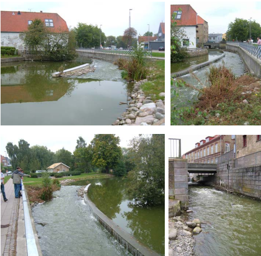
The fauna passage solution on the River Haderslev Møllestrøm showing the outflow from the lake, low-gradient channel, dam wall to retain lake levels but allow flood waters passage, and proximity to buildings and road.
