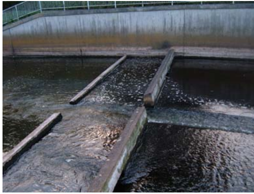
The existing outflow from the pond in the centre of Tønder showing the sloping fish pass channel passing beneath the road from the dam at the other side. Right: The use of low-level concrete baffles to guide fish into the downstream entrance to the fish passage channel.
