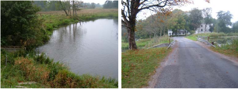
The entrance to the small fish ladder located some distance from the obstacle itself , and the road crossing above the obstacle itself, where a diversion channel will be constructed that will retain wetland habitat upstream but allow houting access.
