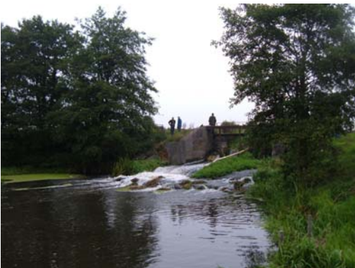
The weir on the River Sønderå (left) created to supply river water to a trout farm downstream (right) currently creates a barrier for fish movement
