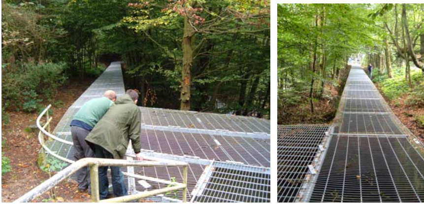
River Varde: The outflow from the lake at the power station. The lengthy step-pool fish way with undershot pipe connectors that currently functions to allow passage into the lake. This fishway would be retained to allow salmon and sea trout movement into the lake.
