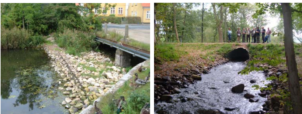
Left: The original exit from the lake used to flow beneath the road and into a mill building. This has been blocked with a new stone weir that retains the lake level but allows high water levels to overspill and prevents flooding. Right: further around the lakeside, a new exit channel has been created and enters the lake just upstream from the new road culvert.
