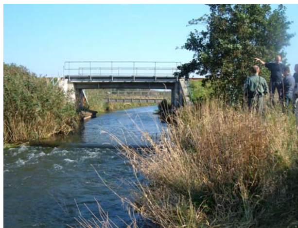
Left: view from weir looking downstream to the staged riffle areas, and right, the original impassable weir now almost fully immersed in water as the downstream streambed has been stepped up to a level just below its crest.
