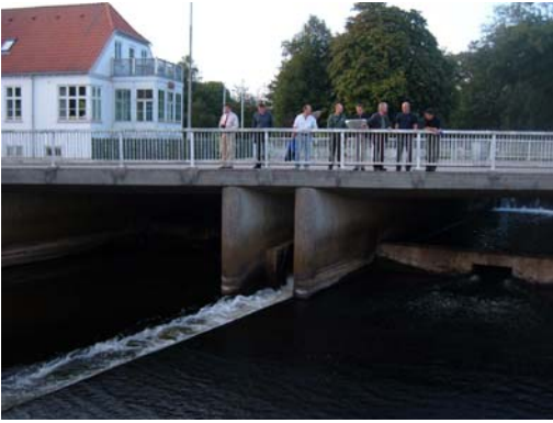
The existing outflow from the pond in the centre of Tønder showing the sloping fish pass channel passing beneath the road from the dam at the other side. Right: The use of low-level concrete baffles to guide fish into the downstream entrance to the fish passage channel.
