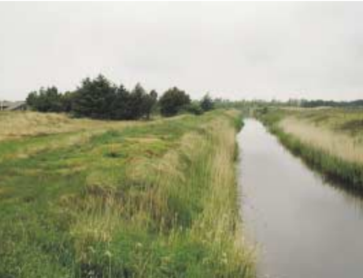
Straightened watercourse with embankments, which effectively stop flooding
